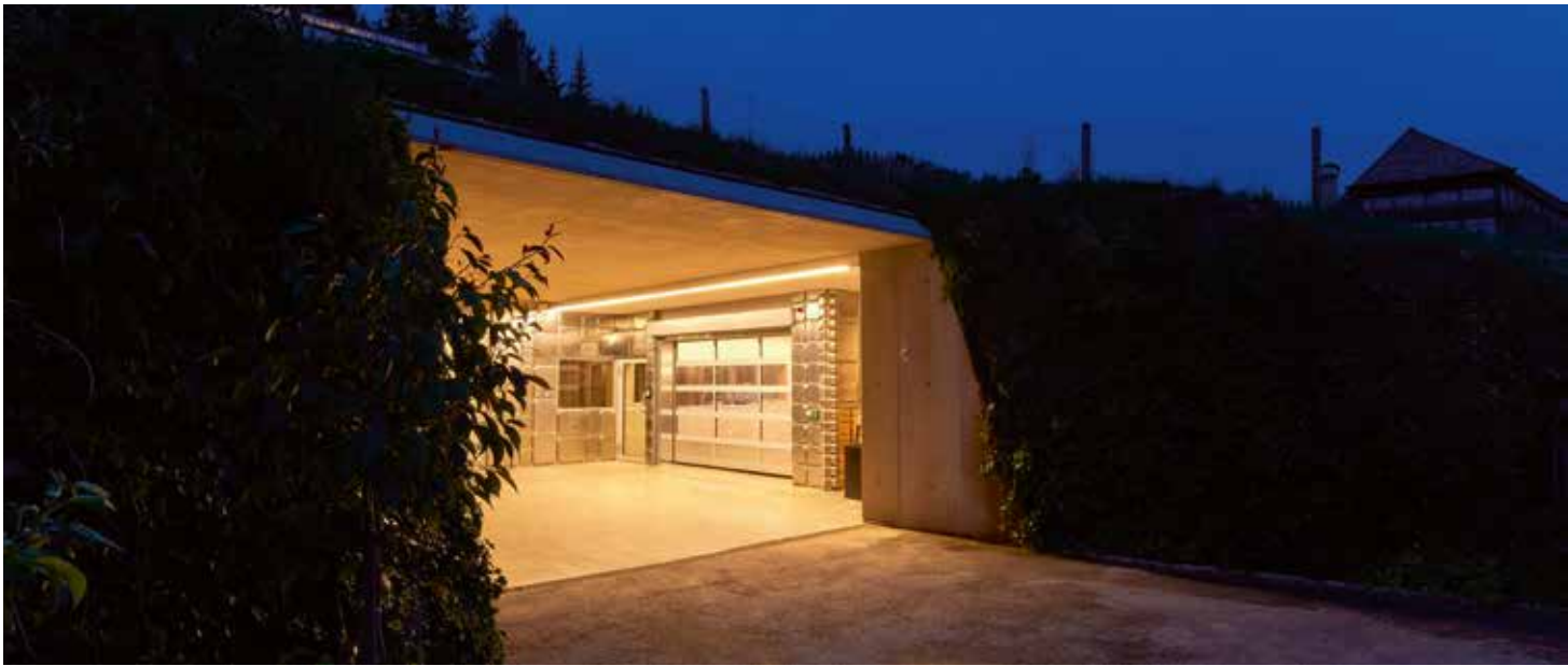
The garage has an open part and a part separated by an industrial sectional door.
