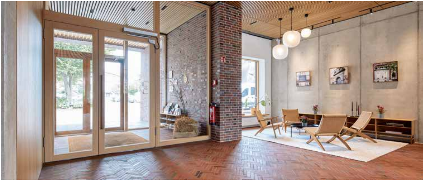
All doors are fitted with automatic closing systems to ensure accessibility.
