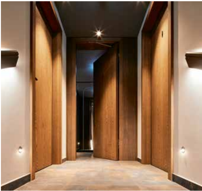
The doors and the timber frame were delivered with a raw oak surface, which the carpenter then finished.
