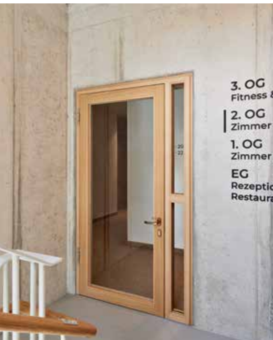
Fire-rated door to the stairwell.
