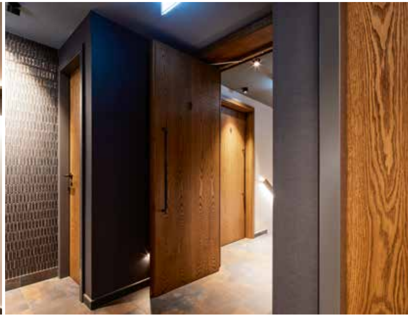
The doors and the timber frame were delivered with a raw oak surface, which the carpenter then finished.
