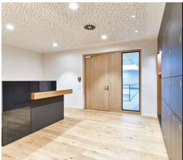
Particularly aesthetic: flush fixed glazing.
