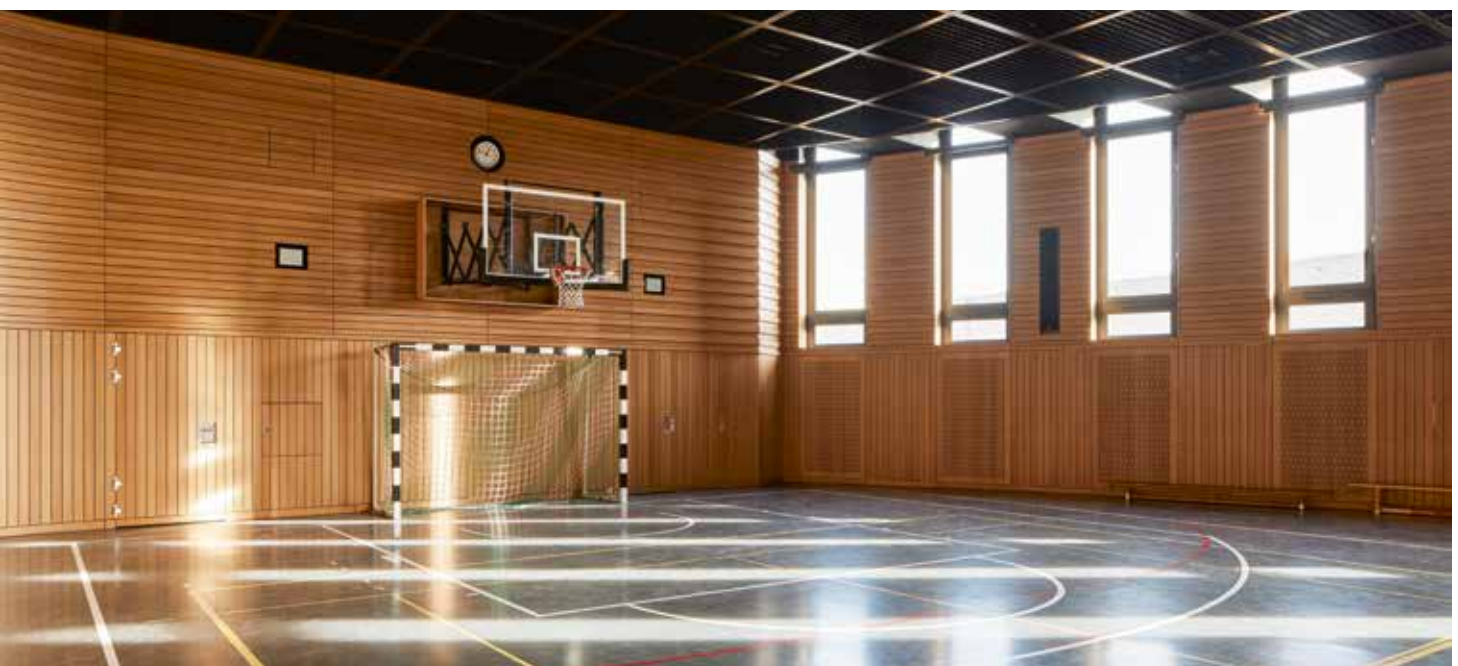
The ceiling and walls also serve as sound insulation. The sound waves should refract on them so that it doesn't get too loud during sports lessons.
