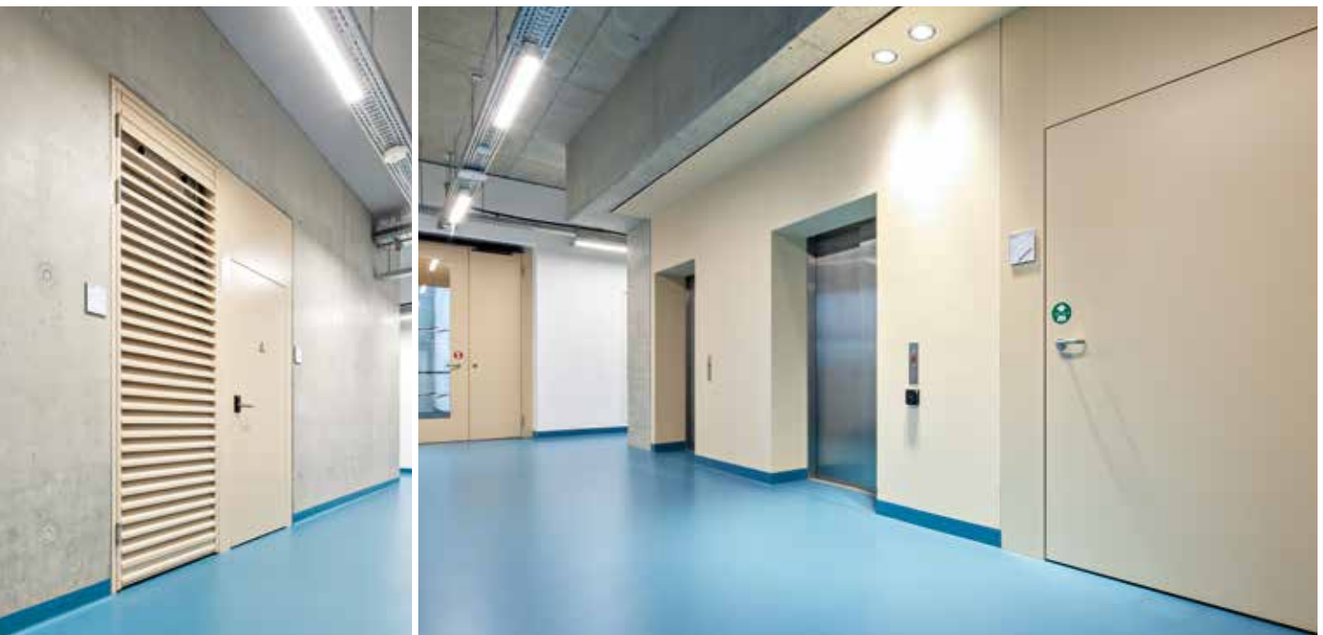
Ventilation slots for technical reasons. The required passage widths are partly ensured by oversized, single-leaf doors.
