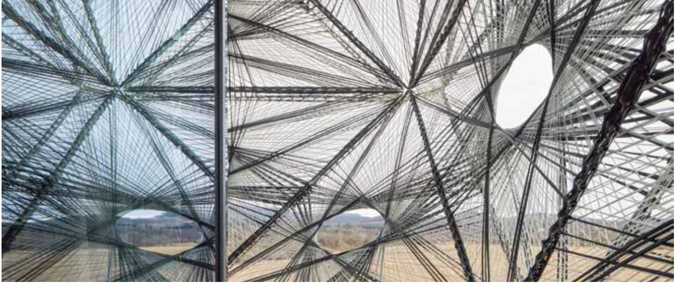
The robotically wrapped façade forms the skin of the Texoversum at a slight distance from the inner façade.
