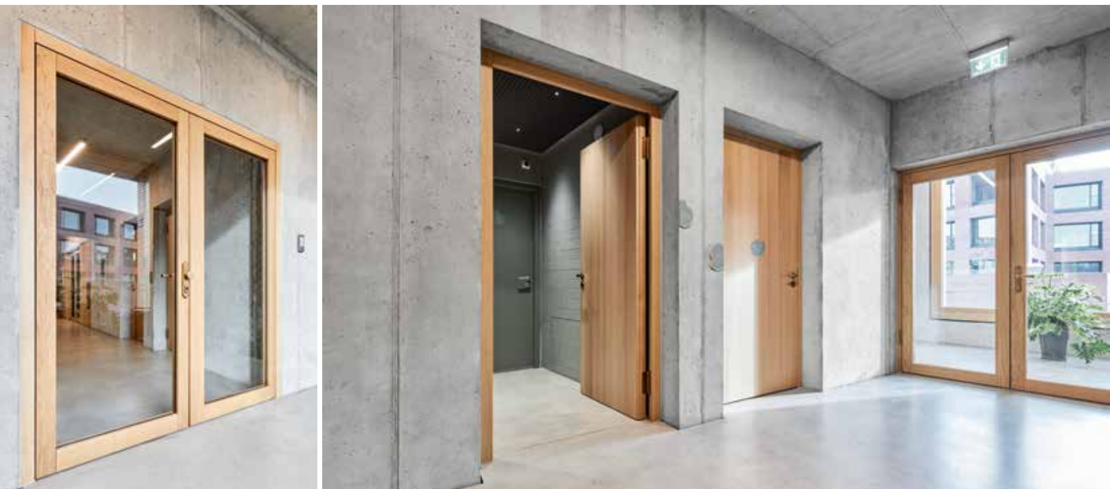
The doors are flush-fitting and flush with the frame and the surface of the wall on one side.
