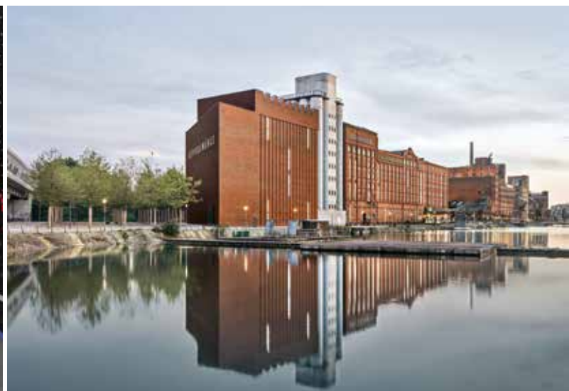
The extension for the Küppersmühle by Herzog & de Meuron.
