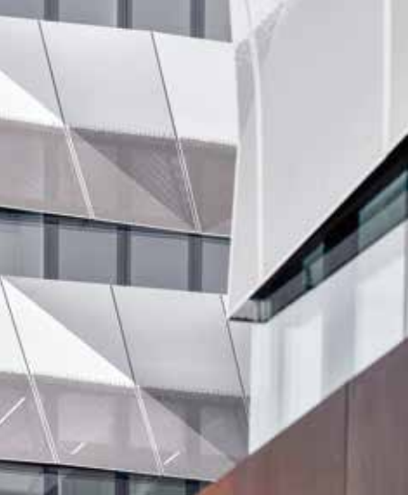
Viewed from a distance, the façade is reminiscent of sails; from close up, the folded and partially perforated metal sheets are recognisable.
