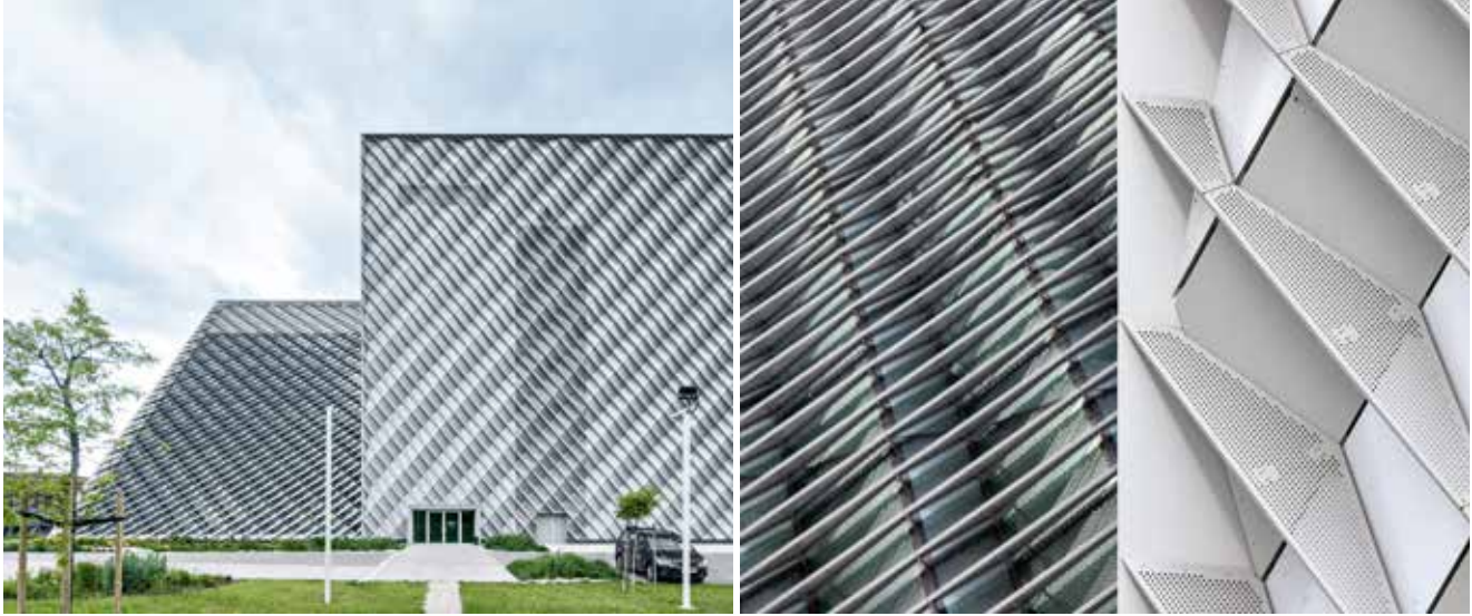
The outer surface is reminiscent of the crystalline structure of a glacier and consists of a multitude of partially perforated metal plates.
