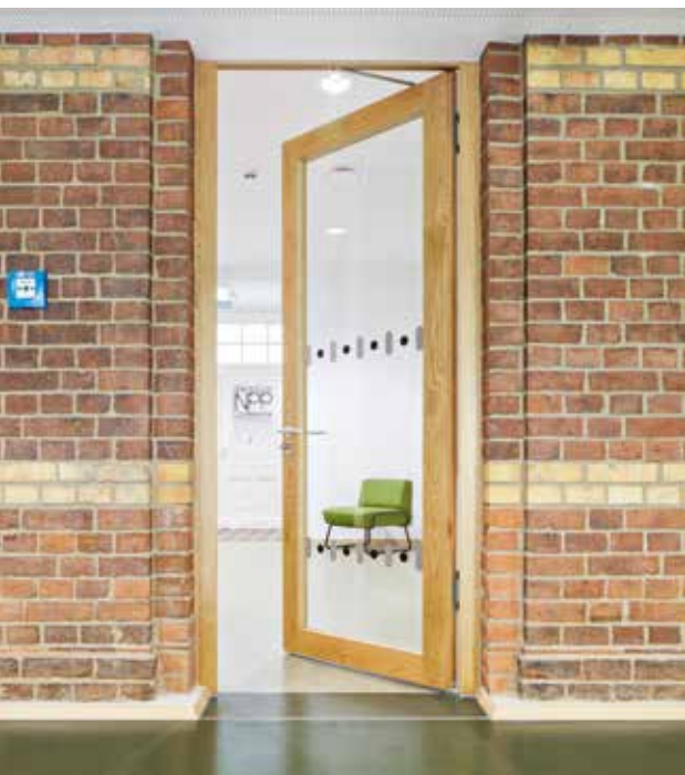
Ceiling-high door at the transition between the old and new.
