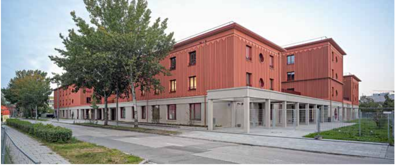
Visually appealing, without being ostentatious: the overnight shelter radiates friendliness and welcomes its residents.
