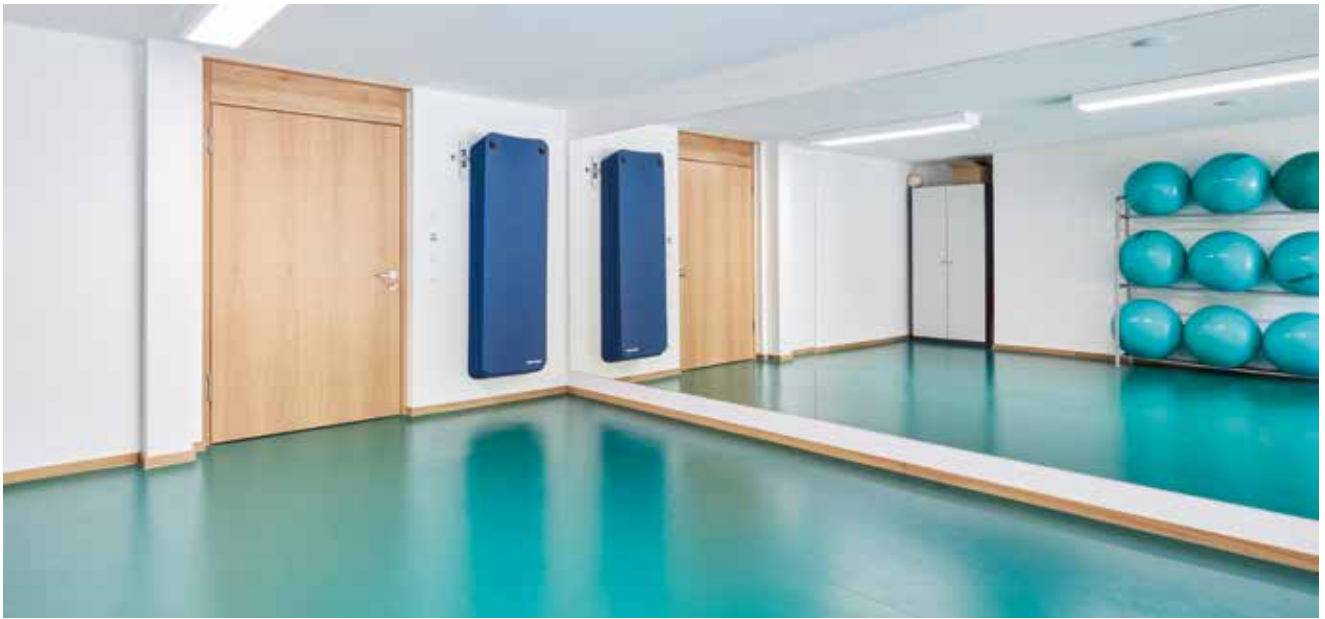
Visually, it is ceiling-high, but instead of a transom light, a transom panel is fitted.
