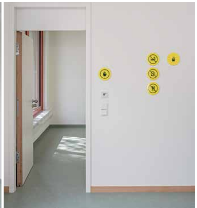
However, some doors are coated in white.
