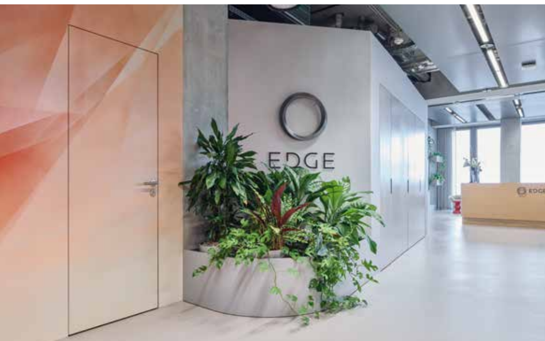
Doors fitted with a zeroline door frame are only distinguishable by the shadow cast by the joint. Depending on the surface, they blend in seamlessly with the wall.
