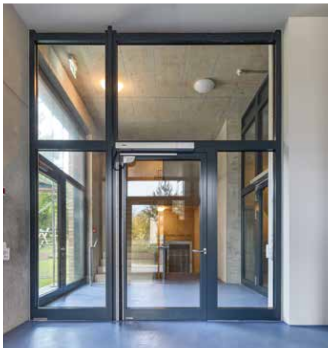
Full-height tubular frame elements form the main entrances.
