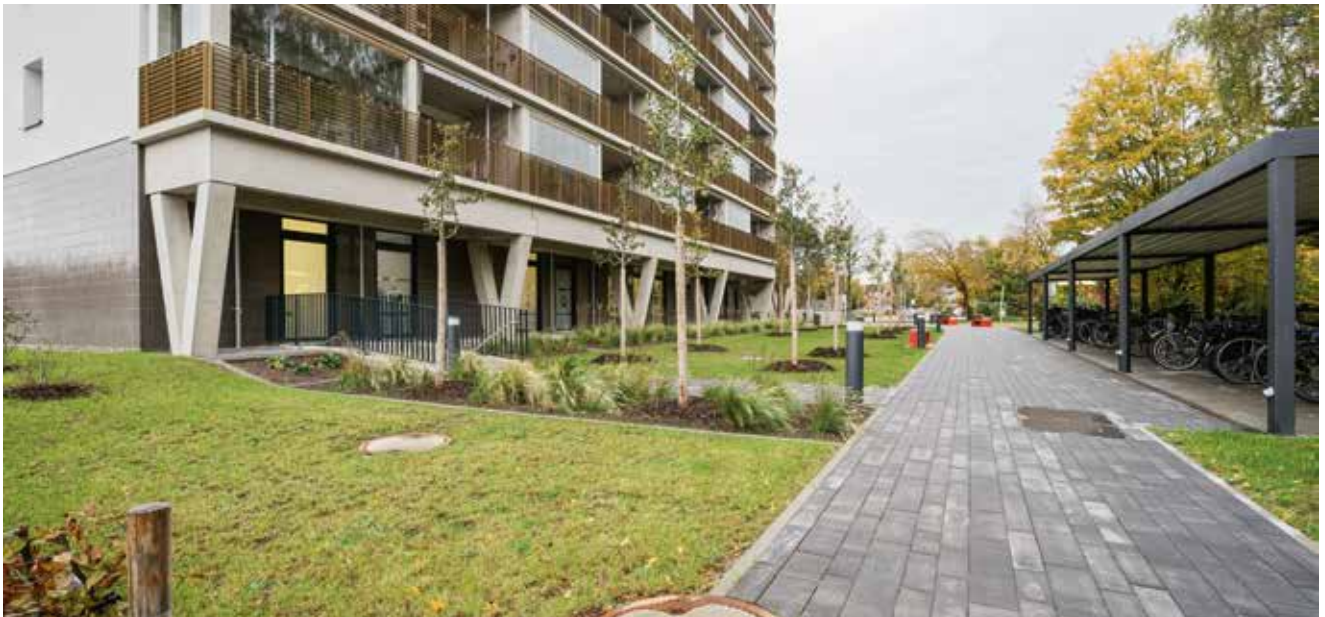
At both ends of the building, staircases lead down to the basement. The rooms immediately behind the doors are used as a bicycle storage room.
