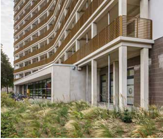
On both long sides of the building, the architects added a self-supporting precast reinforced concrete structure to the existing structure.
