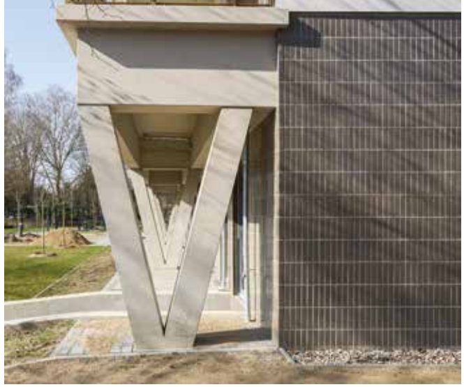
On both long sides of the building, the architects added a self-supporting precast reinforced concrete structure to the existing structure.
